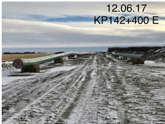
7. Welded and coated pipe on skids – Km 142+400 – Dec 6, 2017
