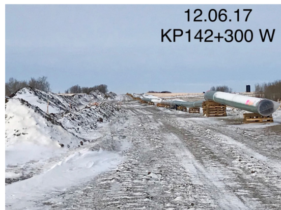
6. Welded and coated pipe on skids – Km 142+300 – Dec 6, 2017
